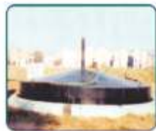
Renewable Energy Biogas Plant
