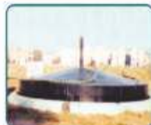
Renewable Energy Biogas Plant
