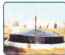
Renewable Energy Biogas Plant
