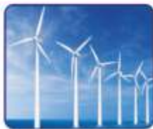
Wind Mill - Capacity 1.25 MW
